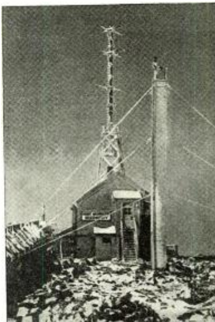
The Mount Washington Observatory, 6,288 feet above sea, atop New England's highest peak. Note the ultra short-wave antenna cross-arms covered with ice.
